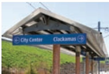
FIGURE 61: Light rail platform shelter
