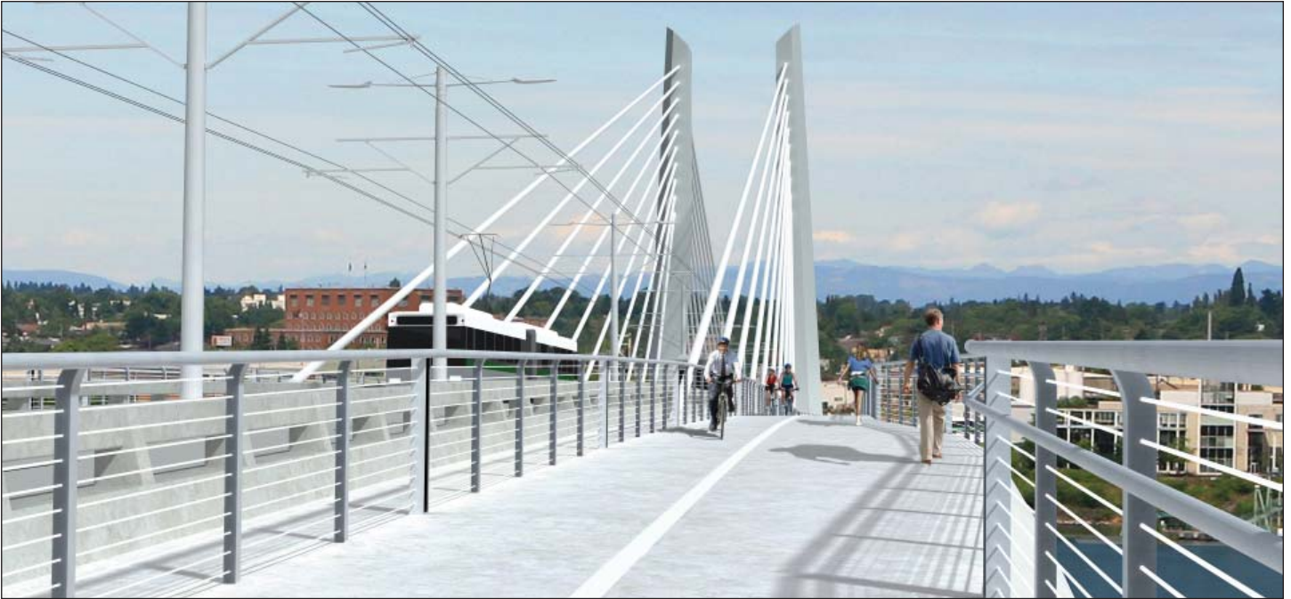
The Willamette River bridge will have 14-foot bike-pedestrian paths on each side of the bridge, as well as belvederes at the mid-span and the towers to allow visitors to stop and enjoy the panoramic views.
