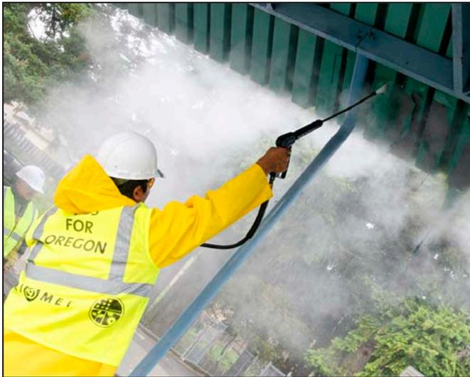
*Crews are stripping the old paint off several Eastside MAX shelters in advance of repainting the stations. The work is funded through the American Recovery and Reinvestment Act (ARRA).*
