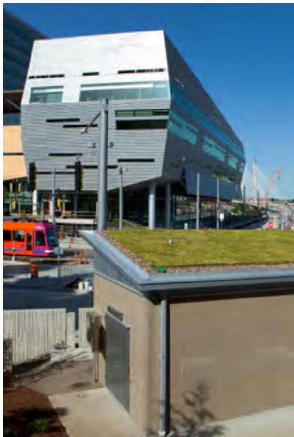
The project includes eight structures with eco-roofs—six on the east side of the river and two on the west side—for a total of 3,500 square feet. Locations include signal and communications buildings, substations and bike facilities. Enviroscapes NW, a Pacific Northwest company, supplied and installed the roofs.
