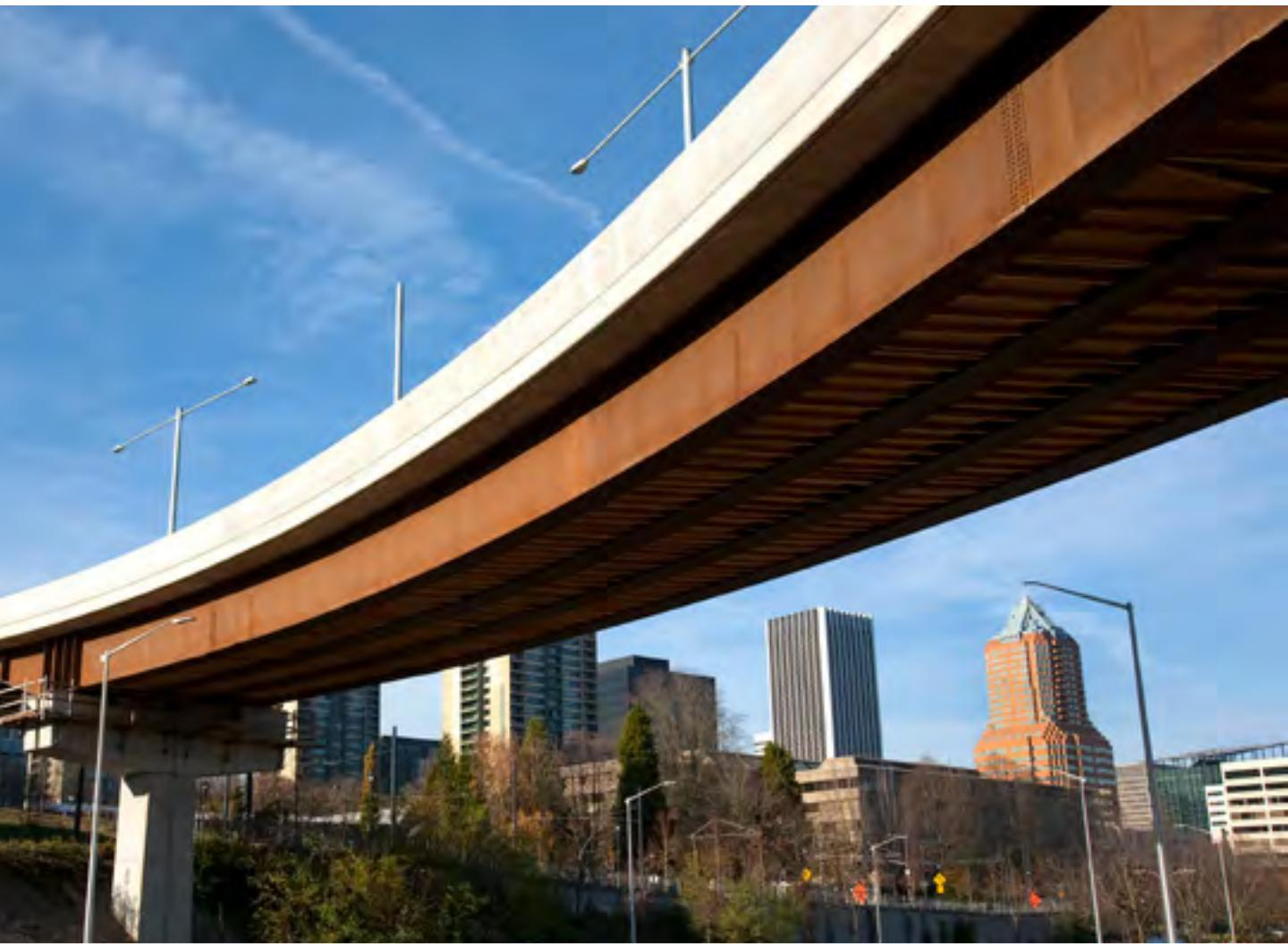
*Low-maintenance materials on the Harbor Structure in South Waterfront include unpainted concrete and weathered steel. The steel girders were fabricated in Tigard, Ore.*
